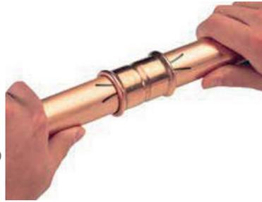
If using slip sockets elongate the V (as per picture) as the depth mark and V can be inserted past this mark.
