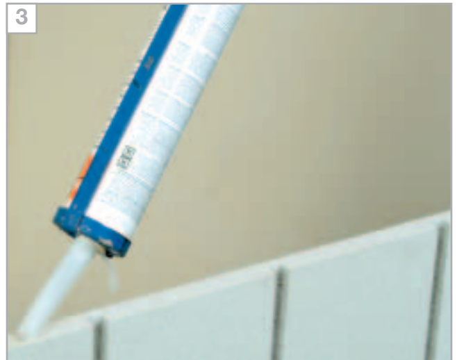
Apply a 3mm bead of adhesive to the end returns of the first panel
