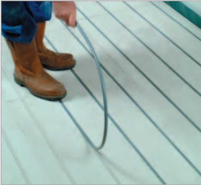
Pipe Installation with Overlay™
