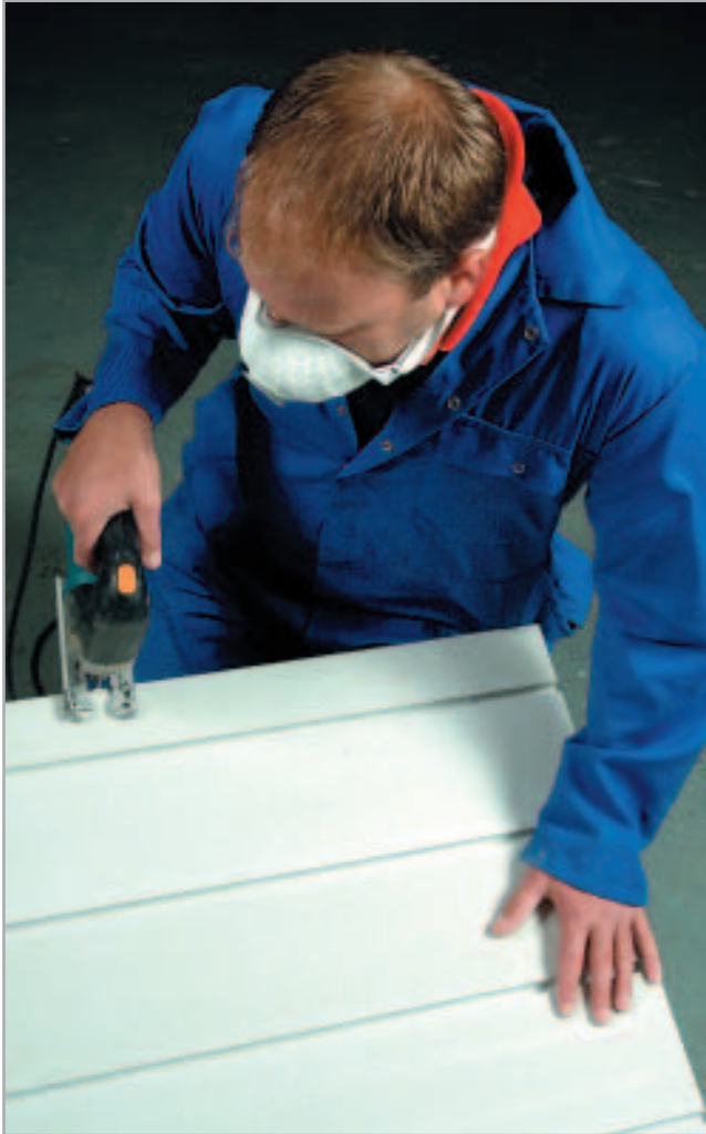
Cut panels using a panel saw, on a low speed setting
